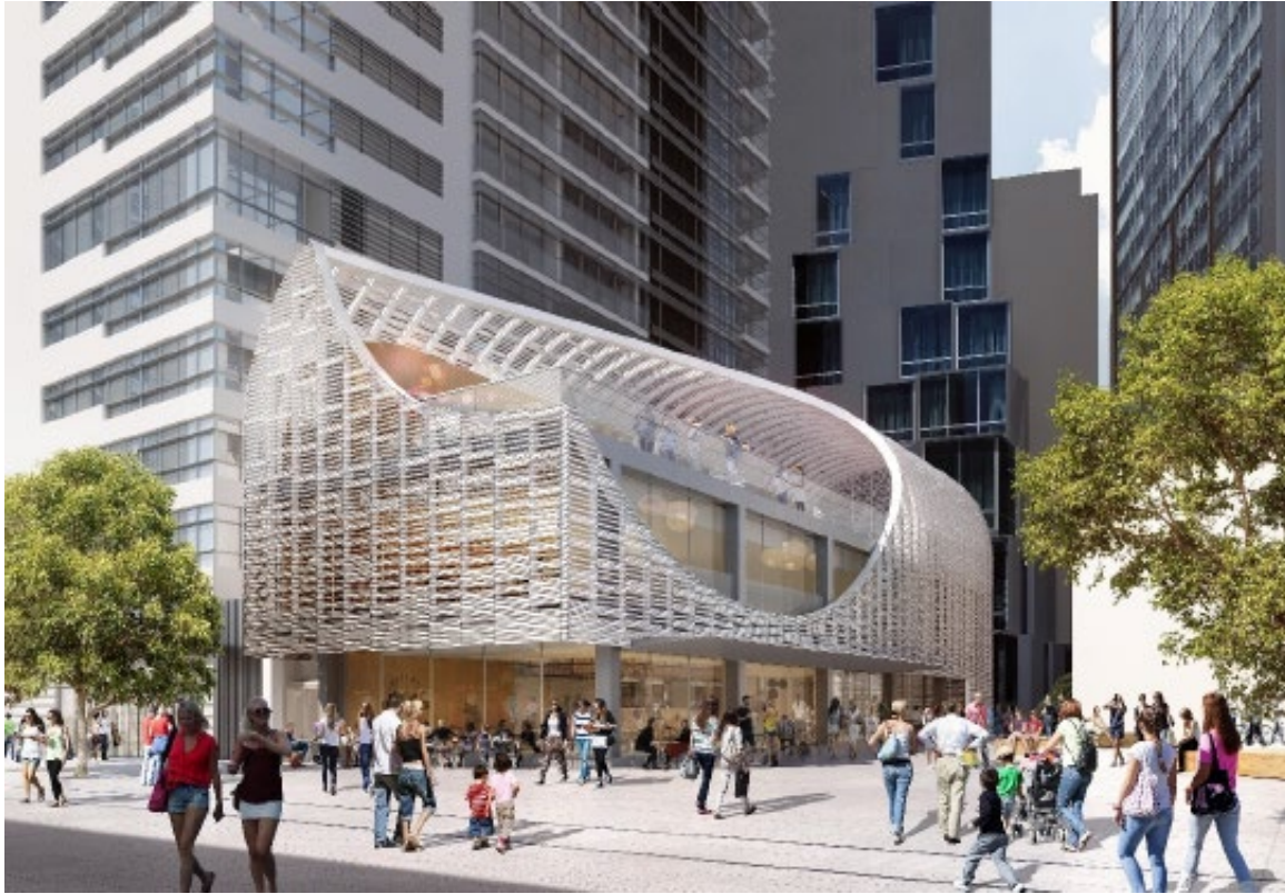
commercial building on Jacksons on George site
